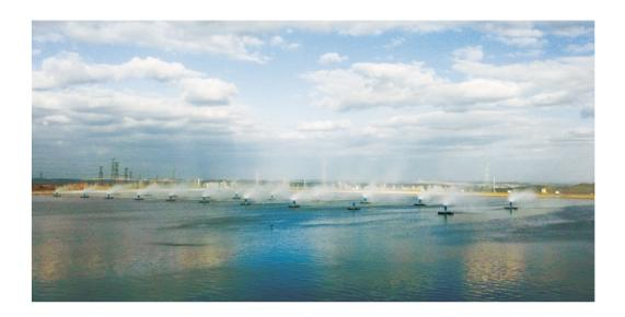
ParKwater® HV10F is a floating mechanical vaporizer, and applicable to small area where wastewater contains large particulates or high corrosion solids. It is reliable, easy to operate and maintain.
